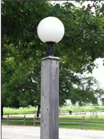
Figures – Examples of current light infrastructure at Middle Fork River Forest Preserve that do not meet the current Dark Sky Program standards.
