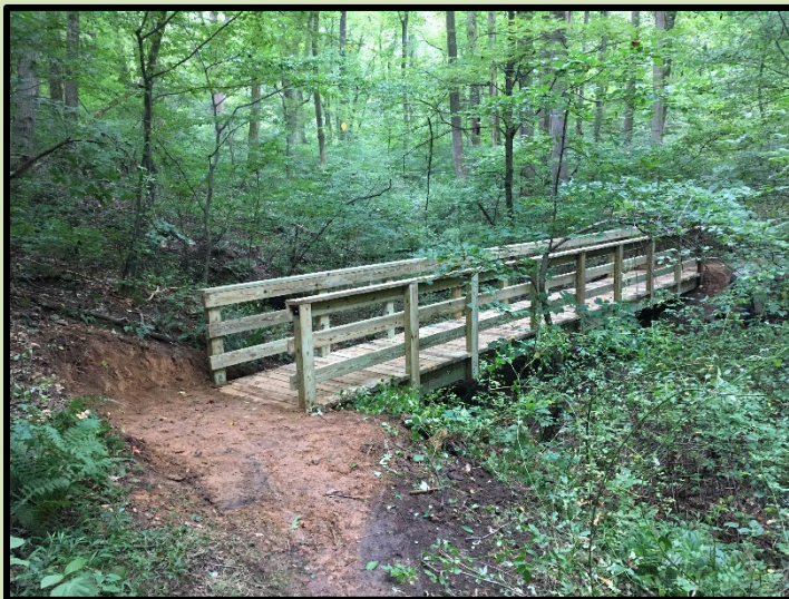
Typical Trail Bridge
