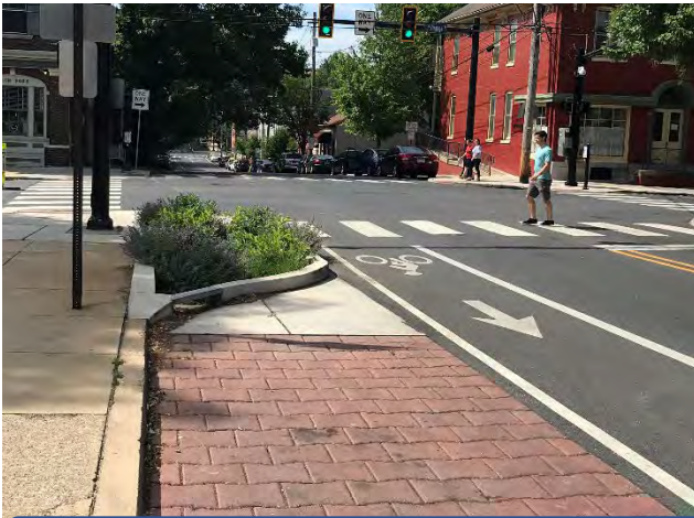
Porous paver parking lanes at Mulberry Street
