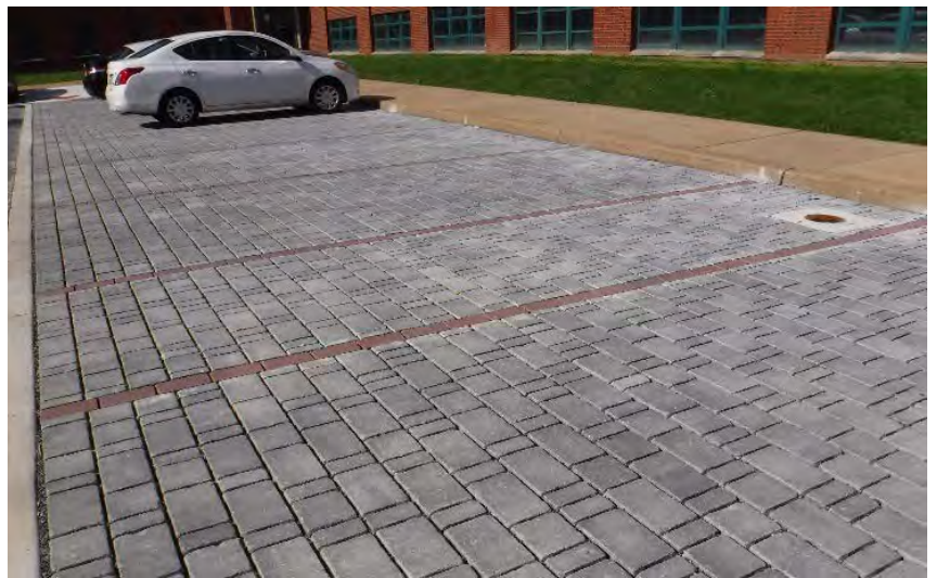
Porous pavement parking spaces, such as these at McCaskey High School, manage school parking lot runoff while improving aesthetics.
