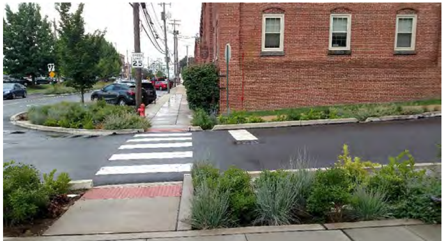
W. Liberty Street features vegetated curb extensions with attractive plantings, new crosswalks, new ADA ramps, and restriped bike lanes.
