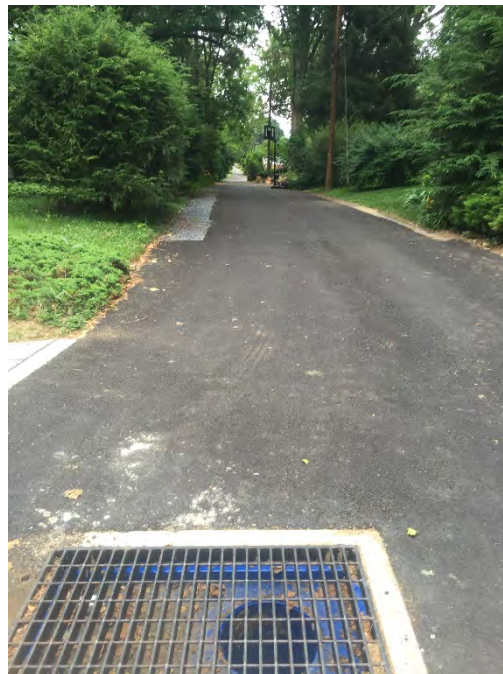
Figure 6.11 – Green Alley Project at Alley 8NW
