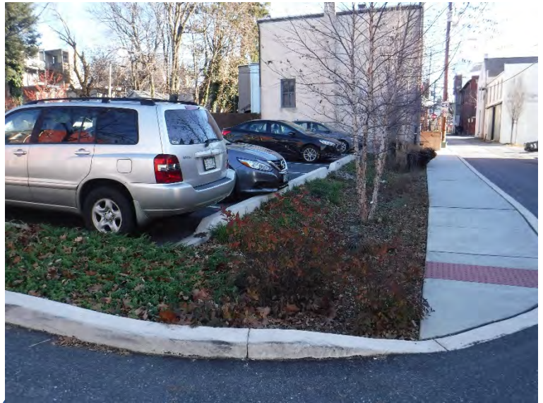
The GI project installed at the parking lot of the Community Mennonite Church features porous asphalt, attractive plantings, and new trees.
