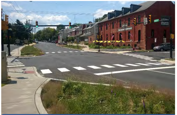
The GI project at Plum and Walnut Streets focused on traffic safety improvements in addition to stormwater capture.
