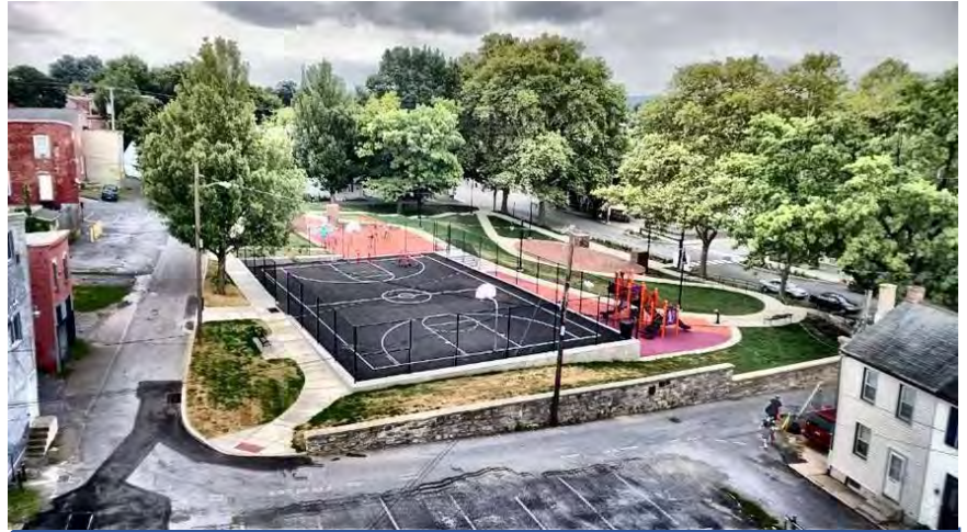
Crystal Park features a porous pavement basketball court, porous paver plaza, and vegetated curb extensions for pedestrian safety among other park improvements.
