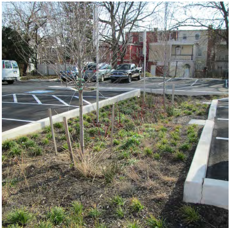
The public parking lot on Mifflin Street features a large bioretention area in the island with native plantings and new trees. The design also featured reconfiguration and restriping of the parking spaces.
