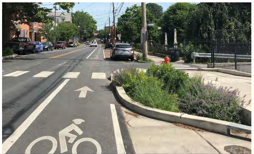
Mulberry Street is an example of a green street project that featured a one-way to two-way traffic conversion and the creation of a dedicated bike lane.
