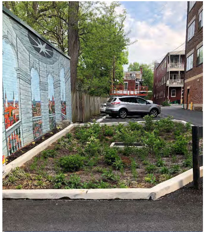
This parking area along North Jefferson Street was reconfigured to include a rain garden. A colorful mural was painted behind the rain garden to add to the overall improvement of the site.
