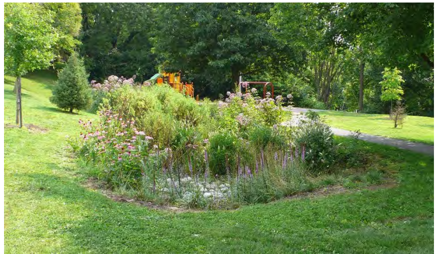
Bioretention areas such as this rain garden at Brandon Park serve to enhance biodiversity and attract pollinators in addition to managing stormwater.
