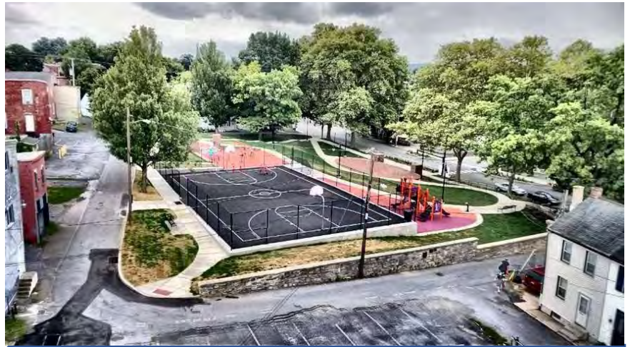
Similar to Crystal Park shown here, Green Schools can feature porous pavement basketball courts and porous pavement play areas.
