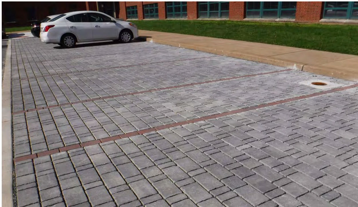
Figure 6.4 - Porous Pavers at McCaskey High School
